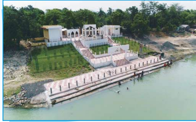
Construction of Sarkanda Bathing Ghat
