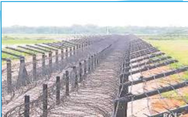
Construction of Fencing Along IBB in Kamalpur, Tripura (work in progress)
