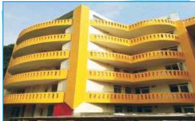
CONCOR, Tilak Bridge
