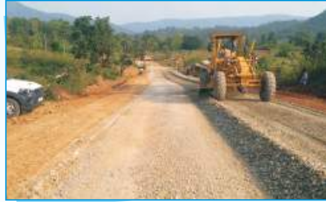
RCD Road Works
