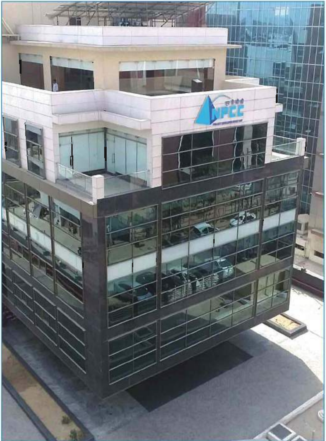
Corporate Office Building, Gurugram
